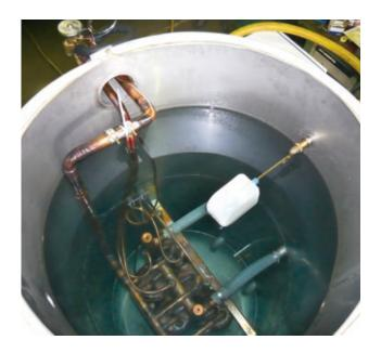
This is an open water system, which is equipped for level regulation with mechanical or electrical filling valves.
